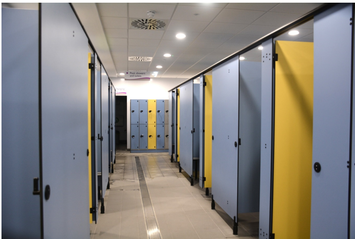
Arundel Leisure Centre – improvements to changing facilities.
